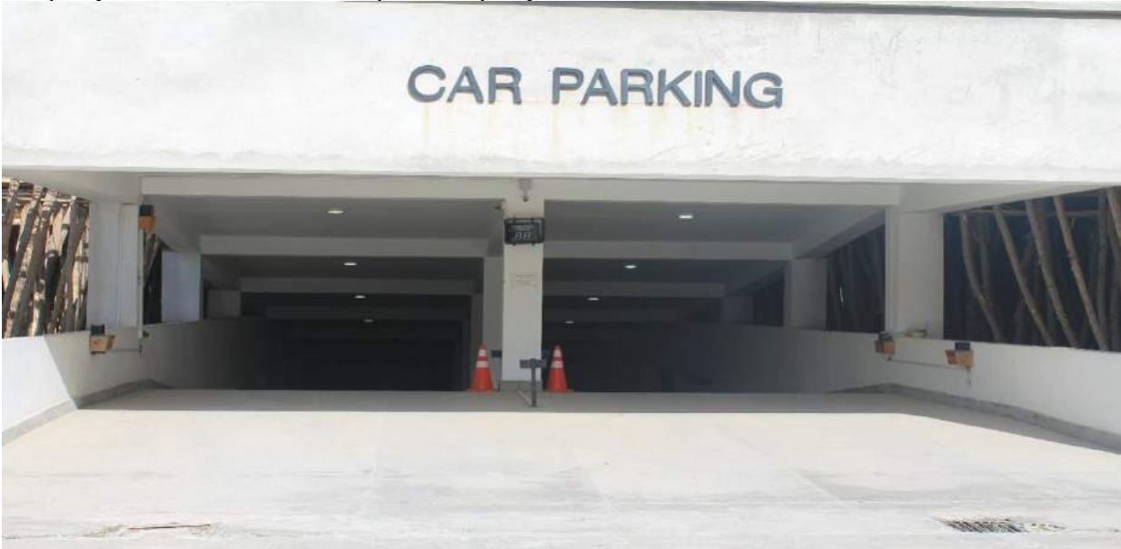
The Opening of the Completed Under Ground Car Student Parking Facility
