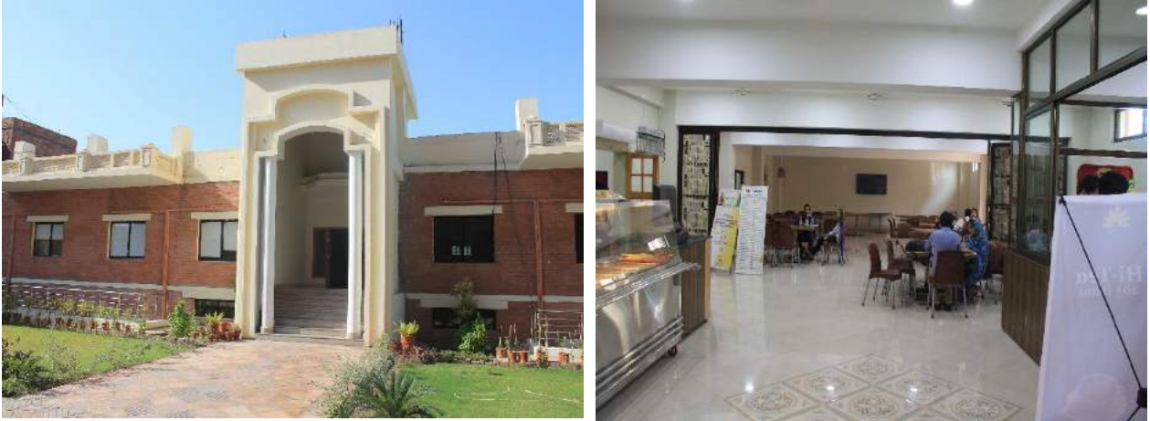
View of the completed Student Teacher Center
