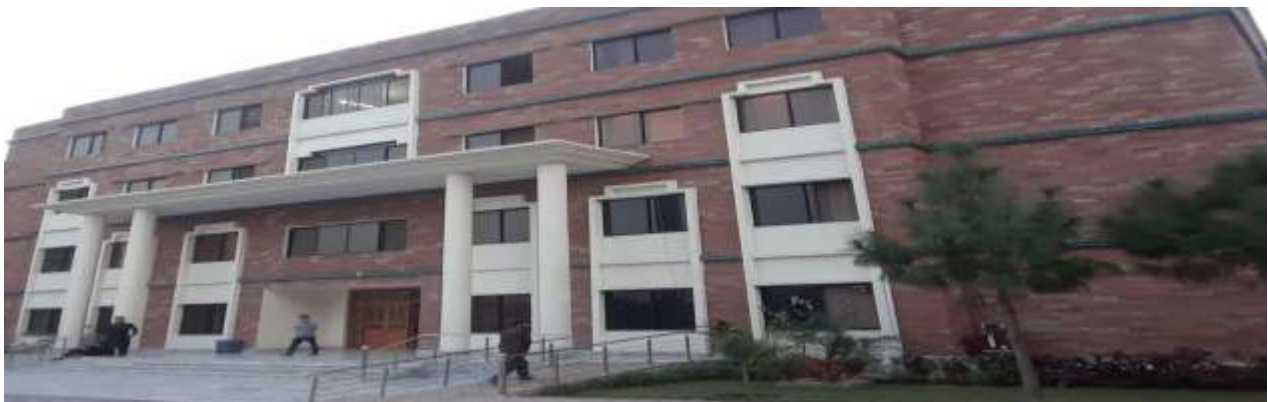
Newly constructed Boys Hostel, IMSciences, Peshawar
